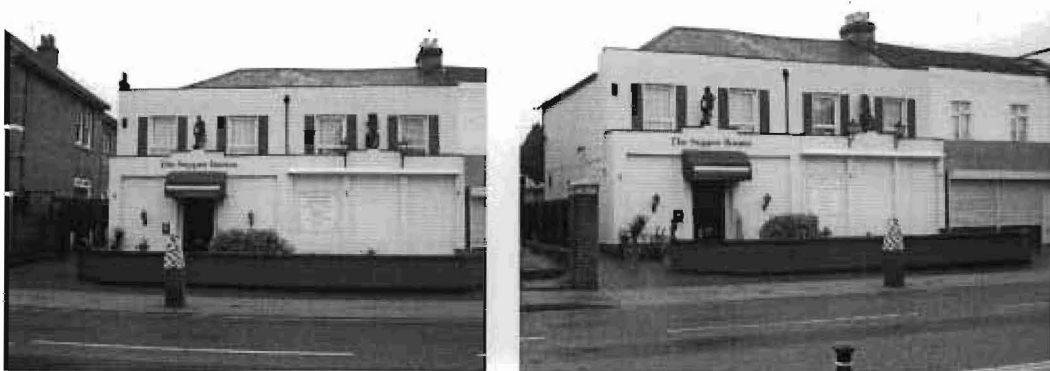
Figures 5 and 6. Application site frontage
